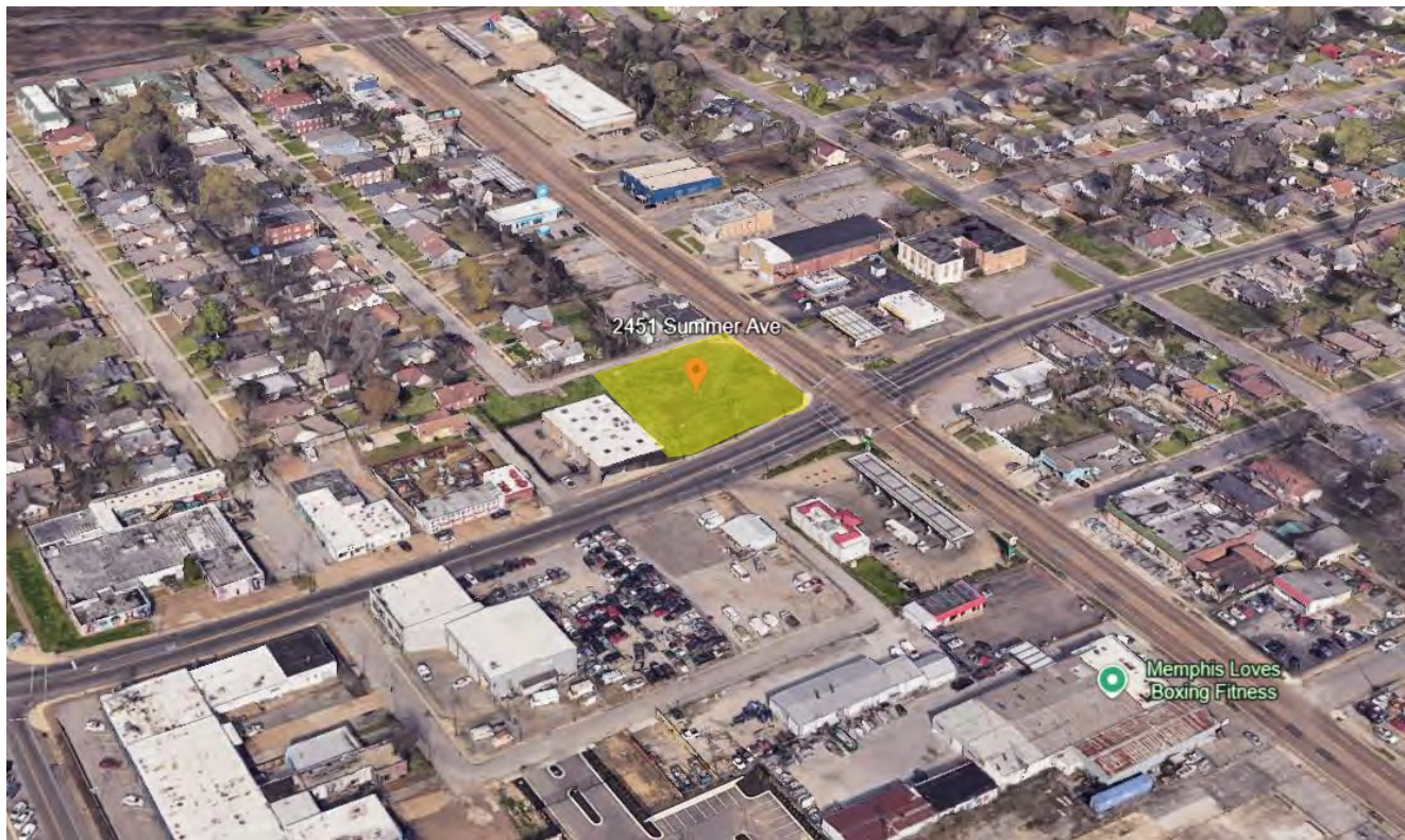
View of subject property from above.
