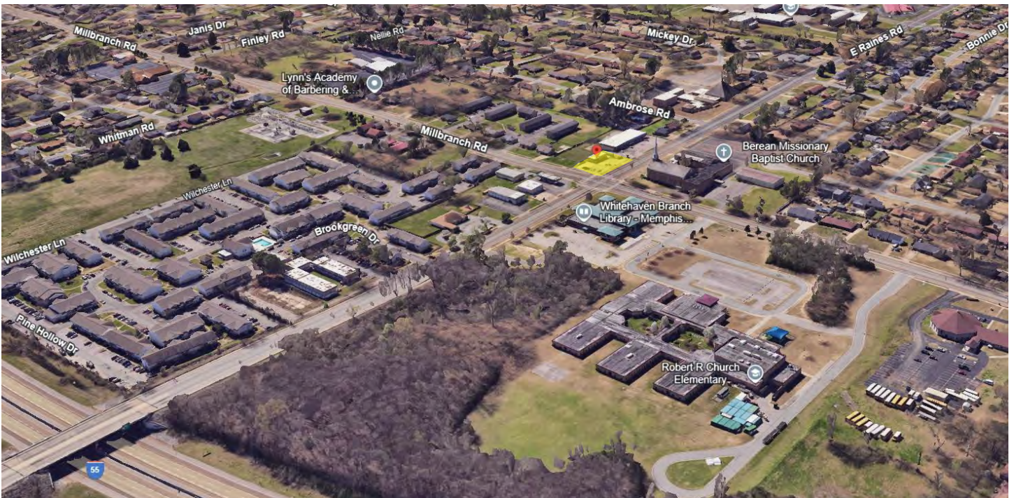
View of subject property from above.
