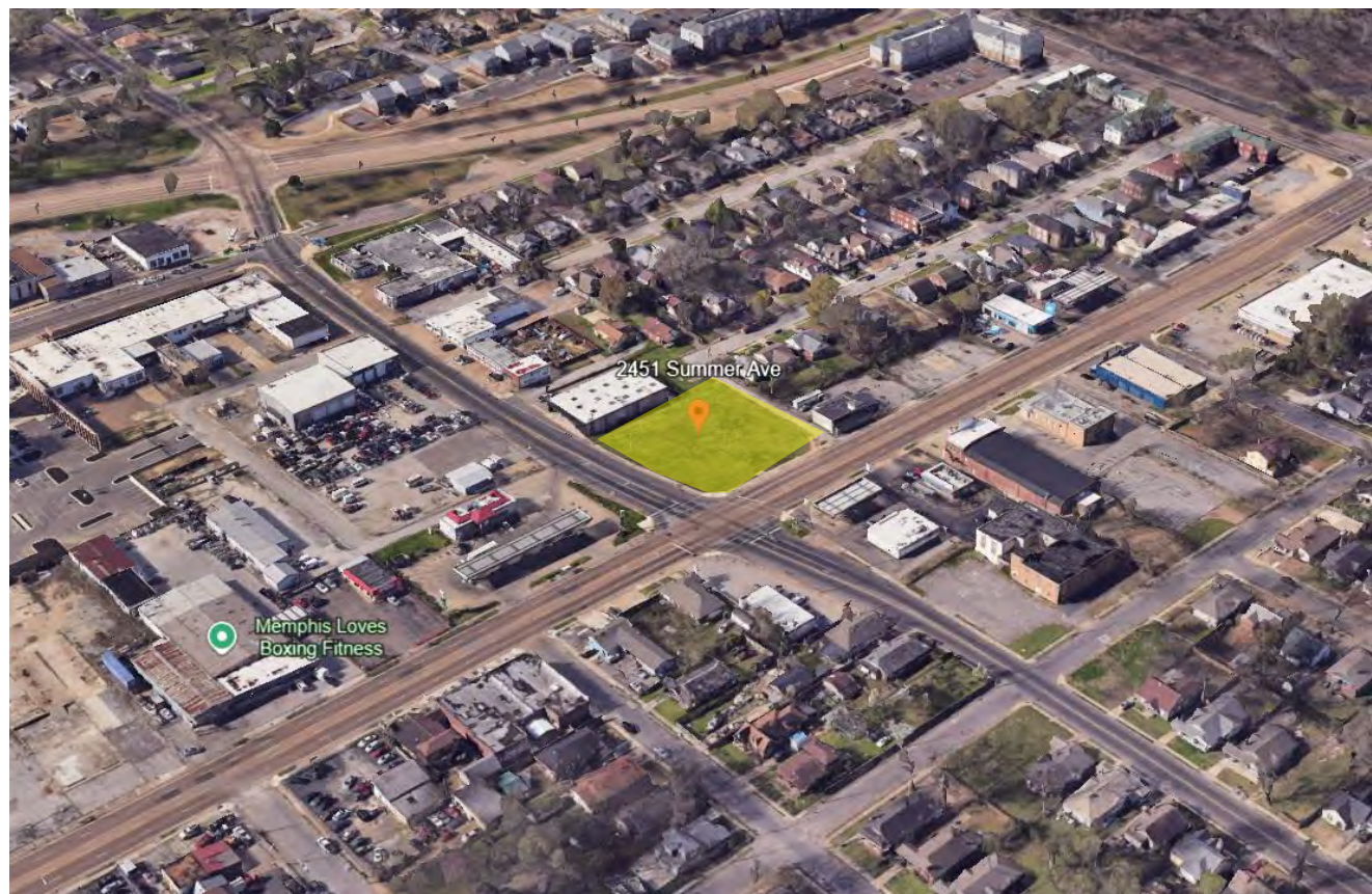
View of subject property from above.
