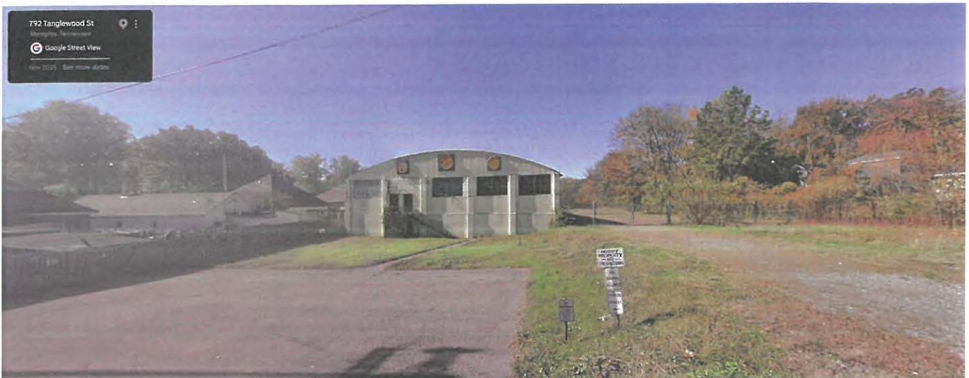
View of subject property from Tanglewood Street looking east
