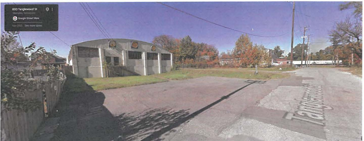
View of subject property from Tanglewood Street looking northwest
