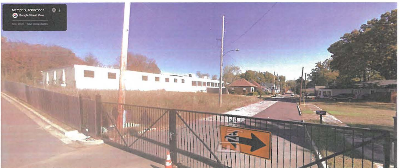
View of subject property from Elzey Avenue looking southwest
