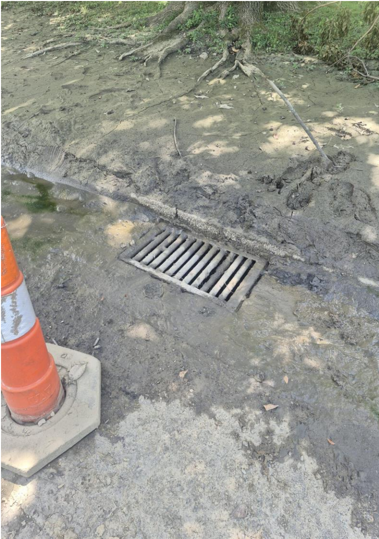
Duck Pond inlet, exposed & cleared
