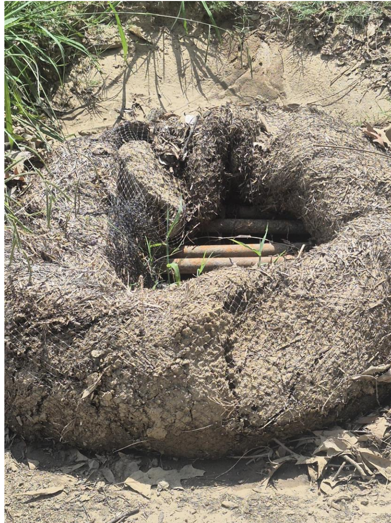
Exposed outlet, cleared (Metal Museum)
