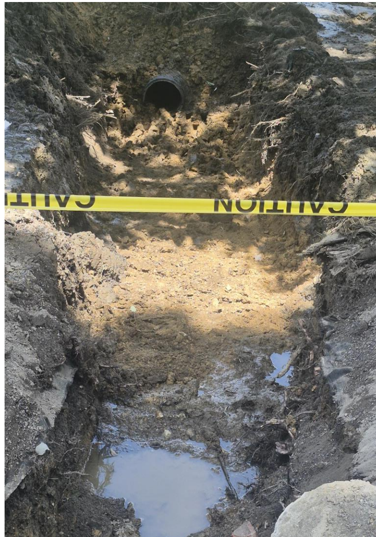
Accumulated mud & debris, cleared
