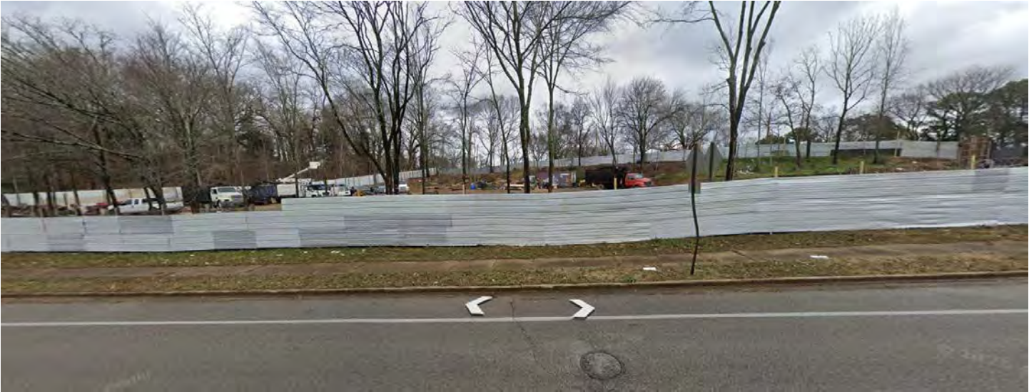
View of subject property from Raleigh LaGrange Road, Dec. 2024
