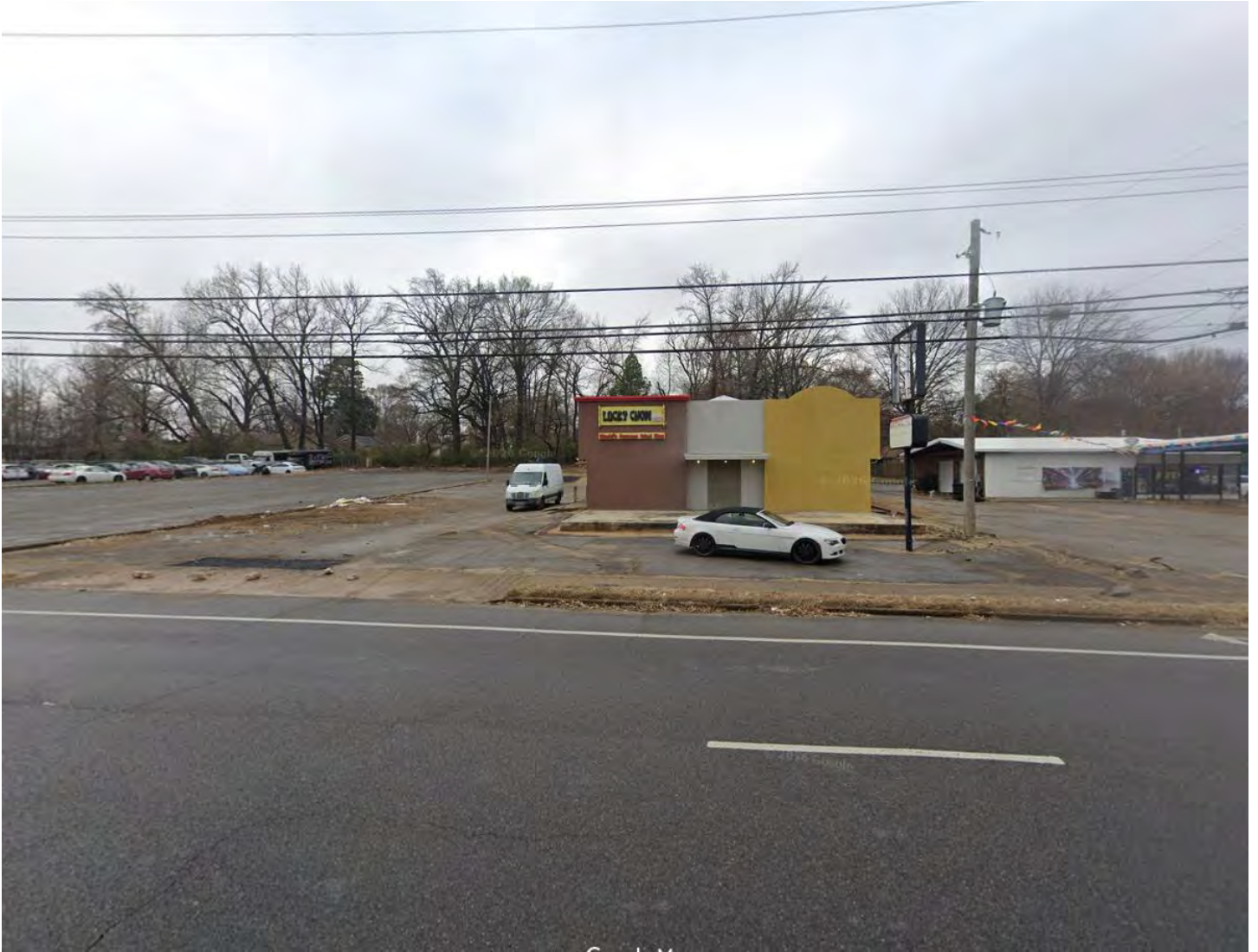
View of subject property from Frayser Boulevard looking northeast
