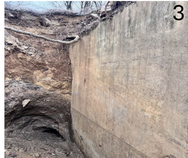
2 & 3 Erosion behind the Right Wing Wall and outside the Wall of the Box.
