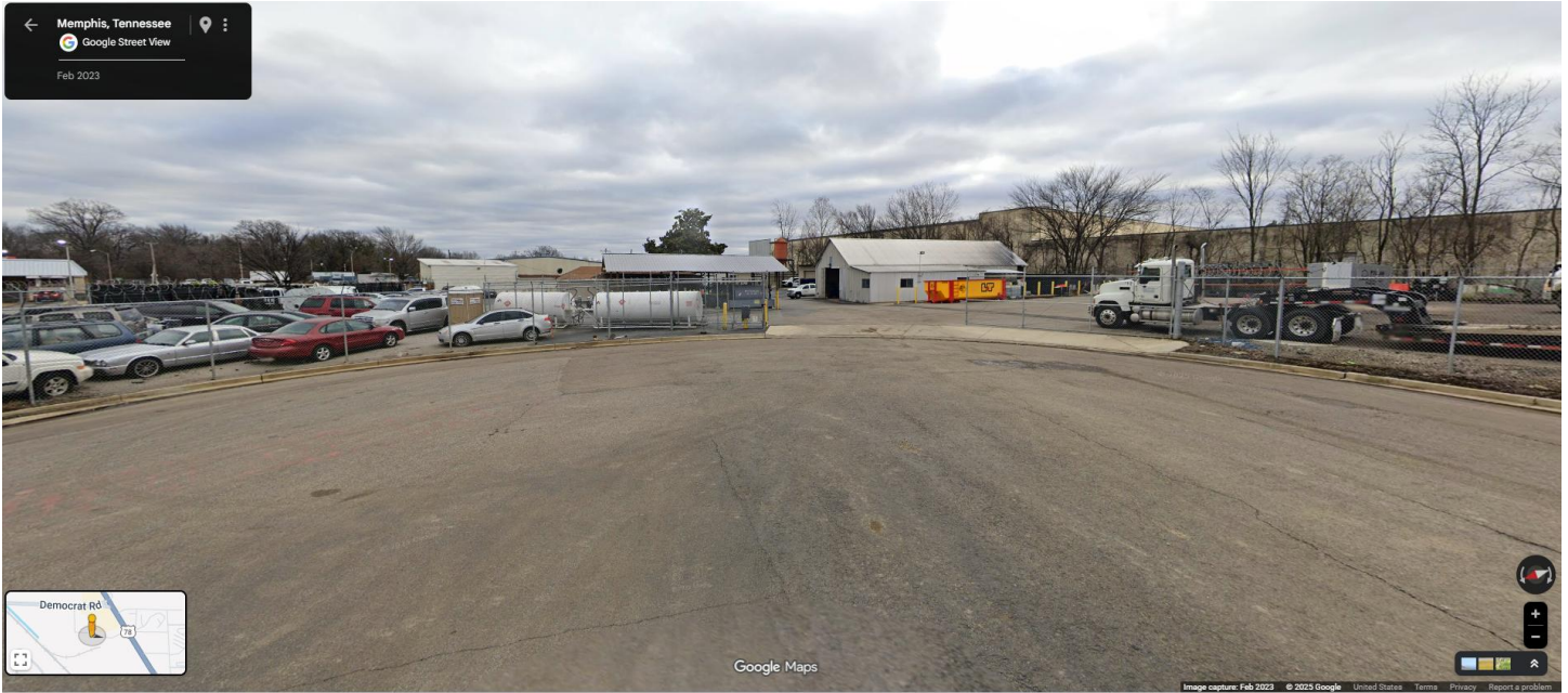
View of subject property from internal driveway looking Southwest
