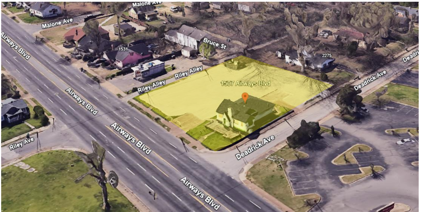
View of subject property from above.
