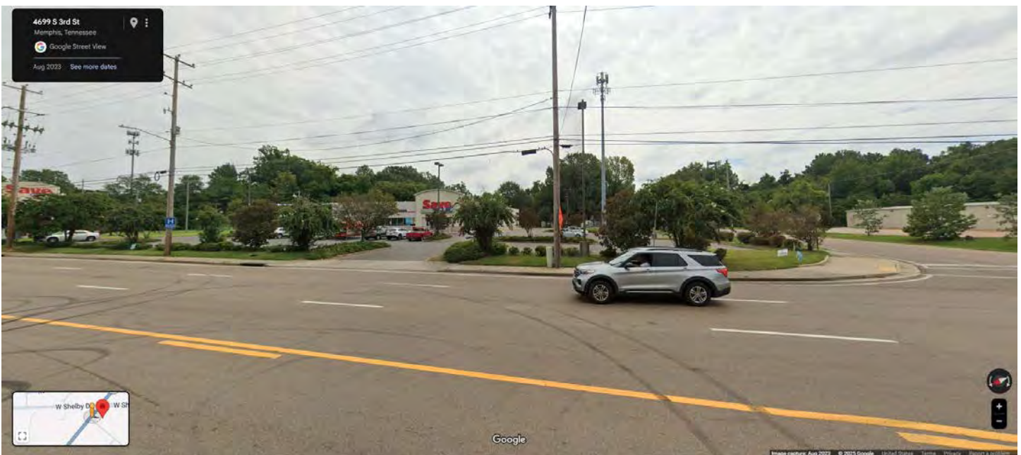
View of subject property from S Third Street looking Northeast
