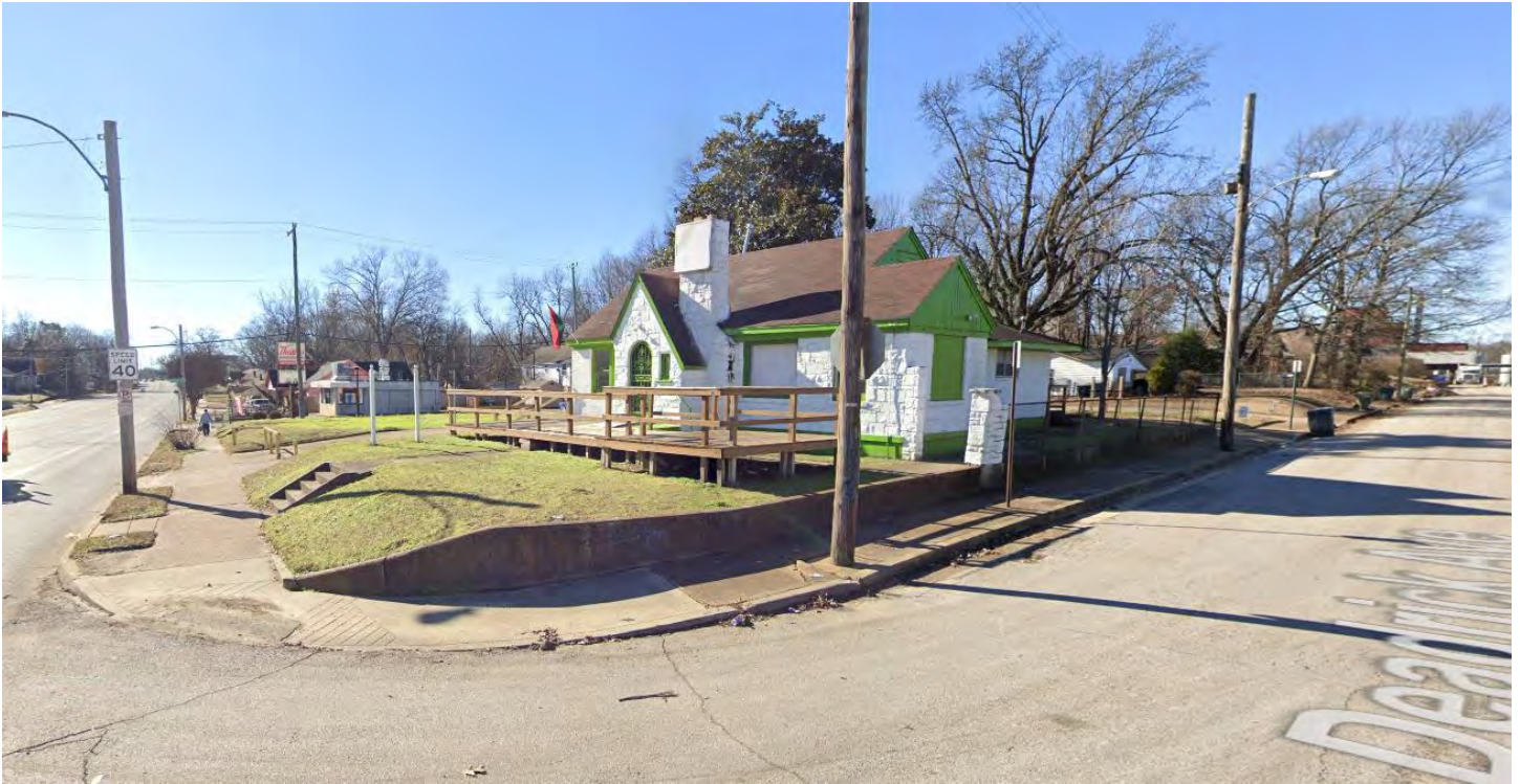
View of subject property from Deadrick Avenue and Airways Blvd (January 2023).
