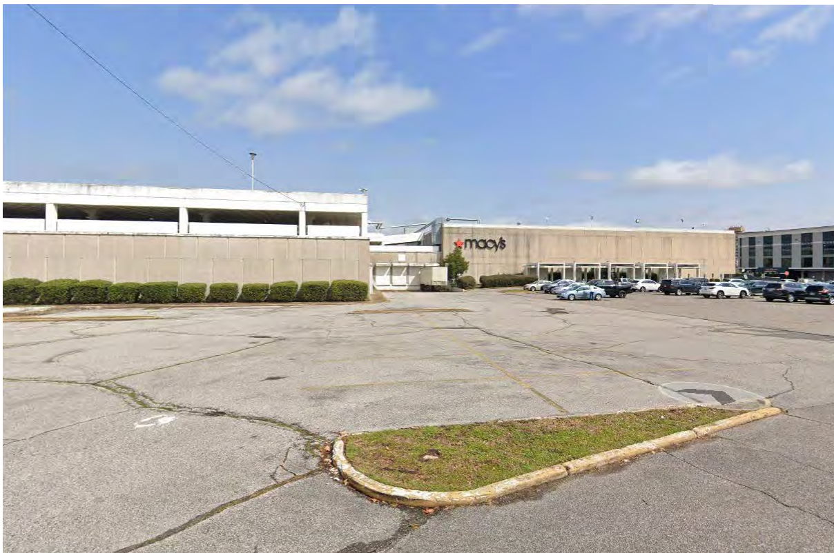
View of subject property from existing southeast parking lot facing north.
