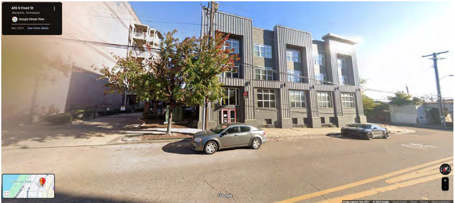
View of subject property from Front Street looking Northeast.
