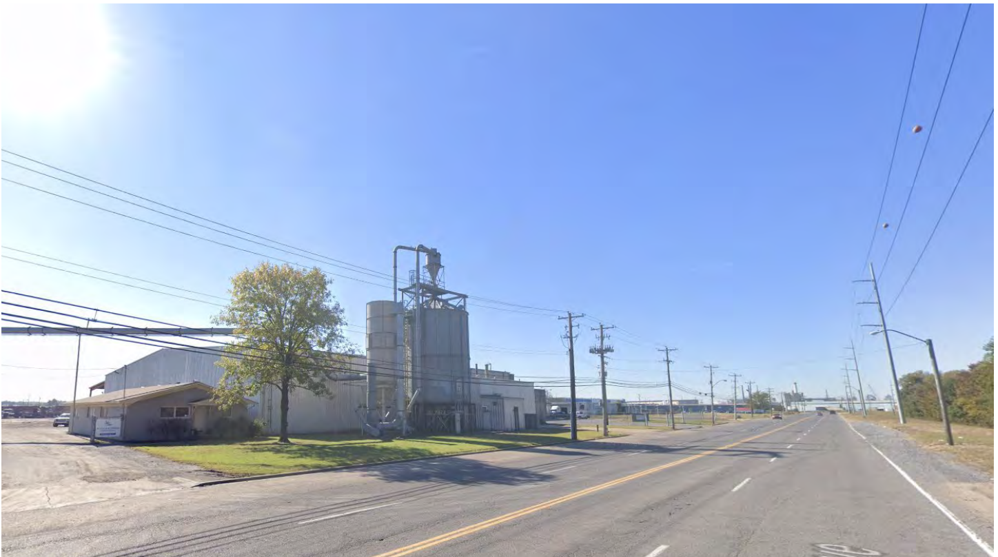
View of subject property from Harbor Ave looking Southeast
