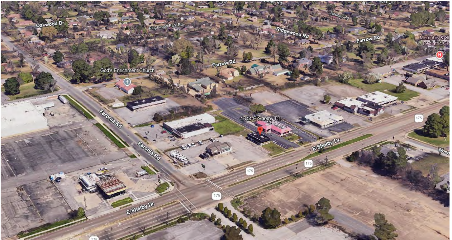
View of subject property from above.
