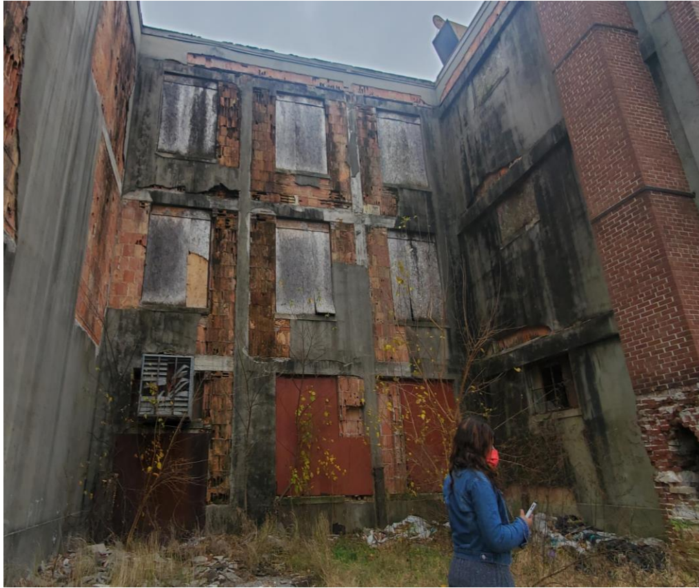
Crumbling back wall repaired
