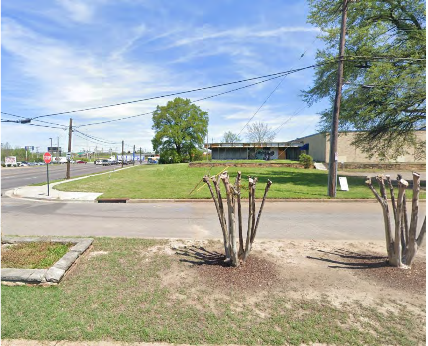
View of subject property from Commercial Parkway looking North.
