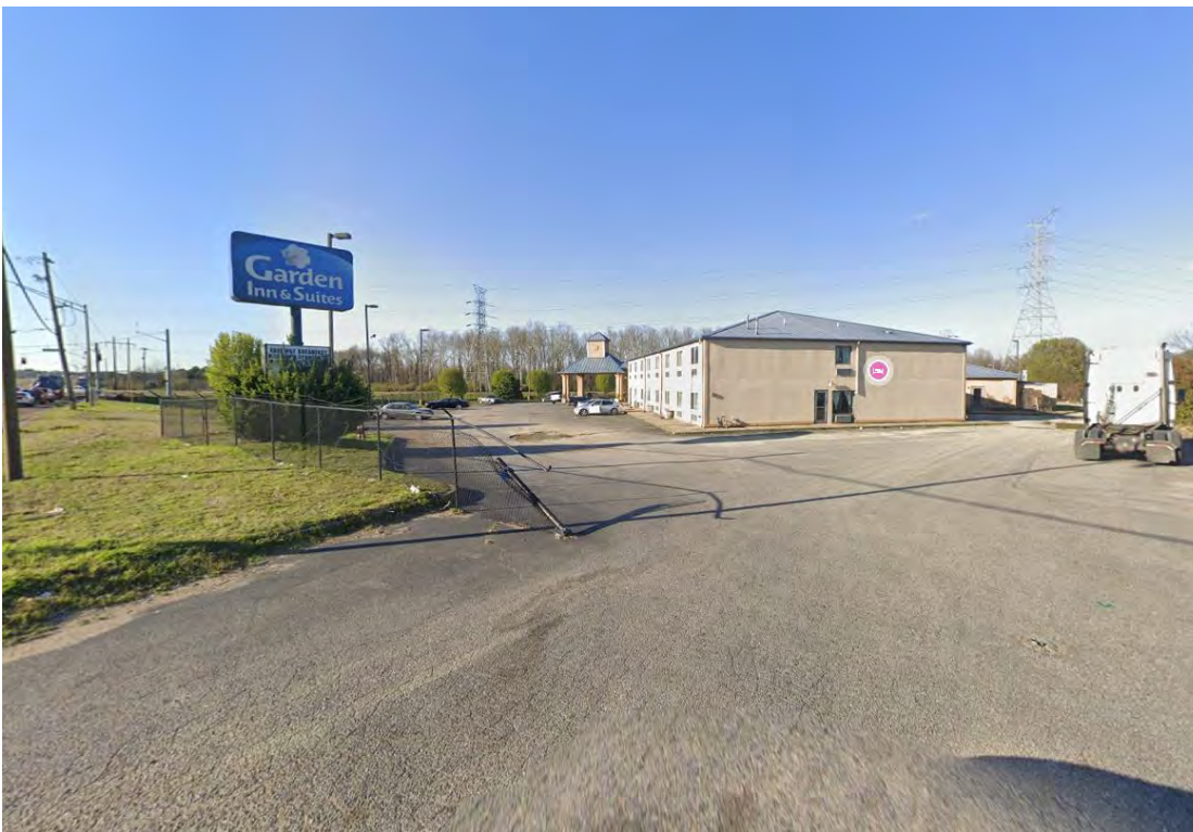
View of subject property from Lamar Avenue looking north
