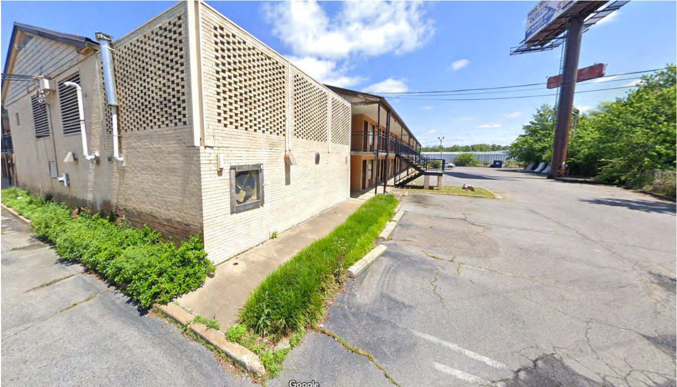
View of southwest corner of subject property.
