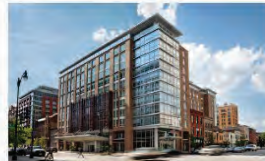
Courtyard & Residence Inn Washington Downtown/Convention Center
