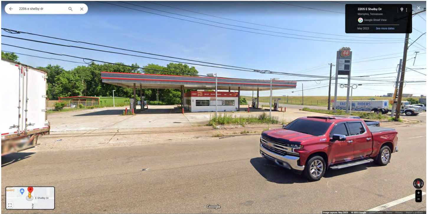
View of existing structure from E Shelby Drive, looking north.
